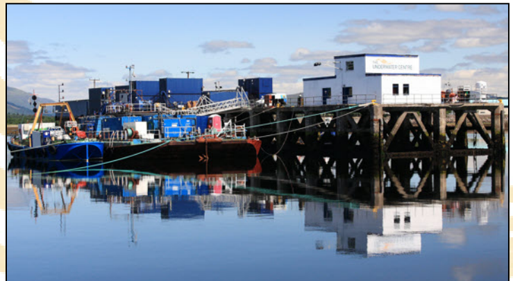
The Underwater Centre's pier facilities stretching out into Loch Linnhe
